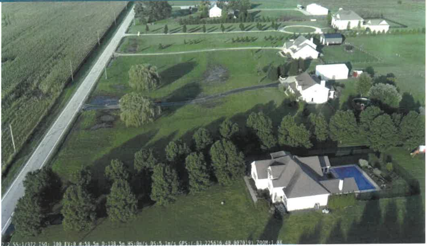
Current aerial photograph of the Patterson Road frontage and surrounding drainage conditions.
