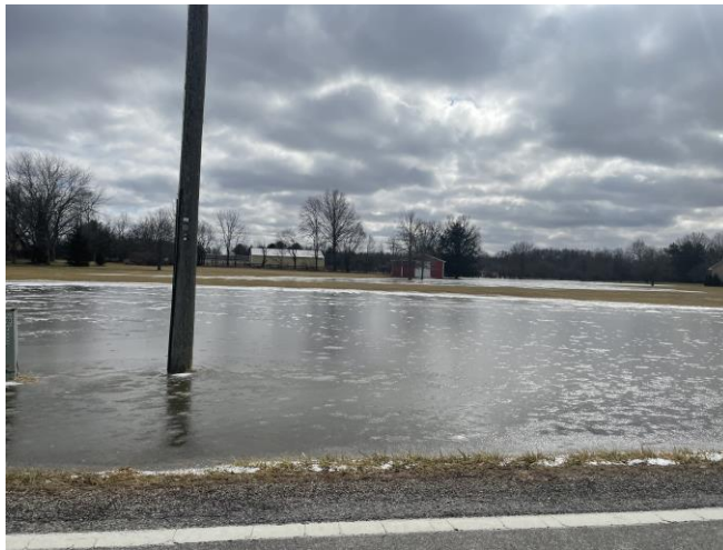
Photo 1 (8669 Patterson Rd. Frontage looking South; Area 1)
