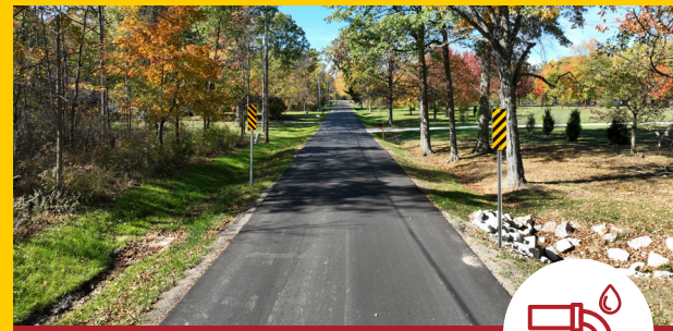
Clouse Road Drainage Improvements
