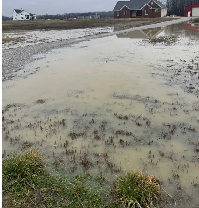
Figure 1: Flooding in the front yard and on the driveway of 4081 Walker Road, built in 2021, facing southwest. This photograph was taken on January 12, 2023 after a 0.88 inch rain event.
