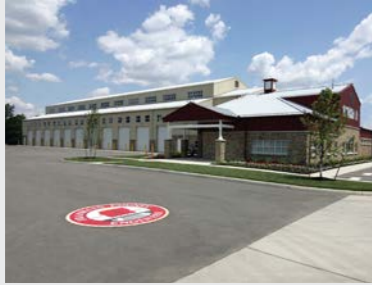
West Maintenance 4444 Fisher Road Columbus, Ohio, 43228 (614) 525-6780
